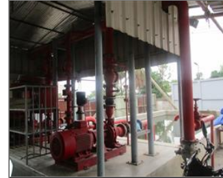
Photo of fire safety equipment Fire Hydrant Pump.JPG
